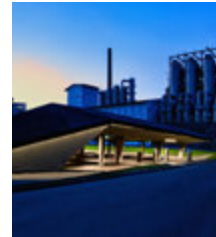
Zeche Zollverein Essen (Germany) Project: Lighting Design: Engineer Büro Paulus Essen, Herr Gräf
